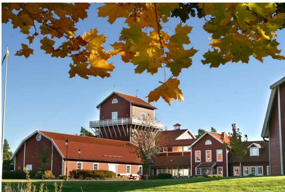
Figure 2 Surface buildings of the SKB Åspo Underground Rock Laboratory for radioactive waste management research near Oskarshamn Sweden (Source: SKB)
