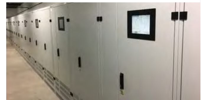
Inverter and DC cabinets
