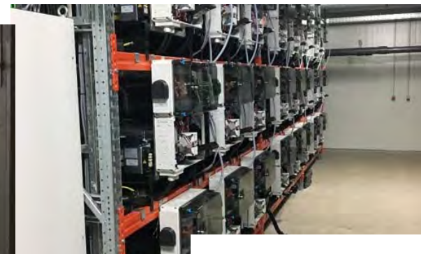
Inverter and DC cabinets
