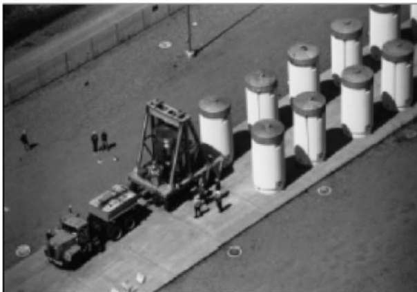
Figure 2.2: Concrete storage casks at a U.S. nuclear power plant
