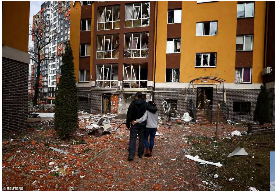
A couple hug each other while walking beside a building damaged during the shelling amid Russia's ongoing invasion of Ukraine, in Irpin, Ukraine March 31, 2022.
